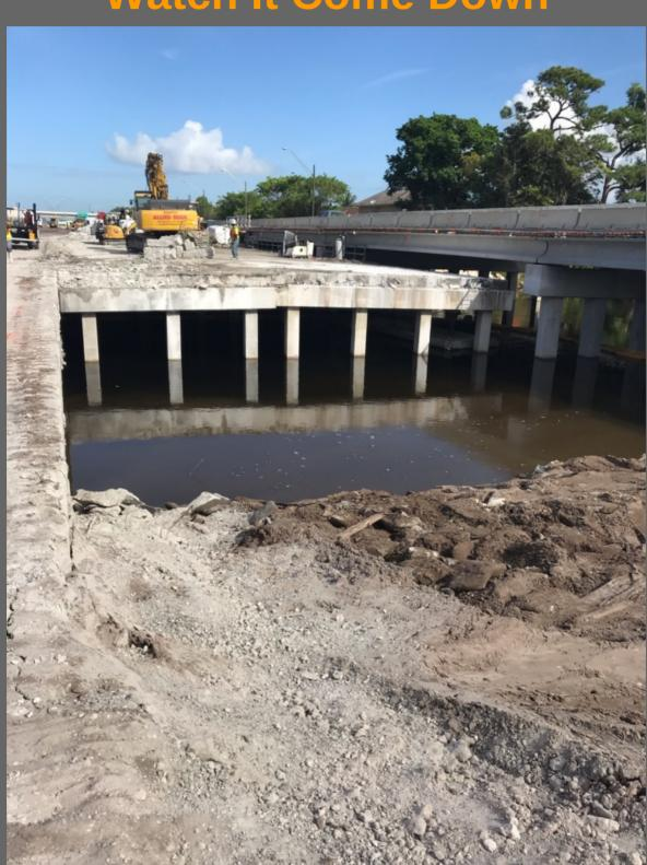
the Alliedbean crew successfully removed the deck, pier caps and piers of the 26,800 SF bridge located on I-95 and Hillsboro Boulevard in Broward County, FL. The removal of this bridge has a very unique set of challenges being an active waterway below and a fully operational expressway that cannot be disrupted.
