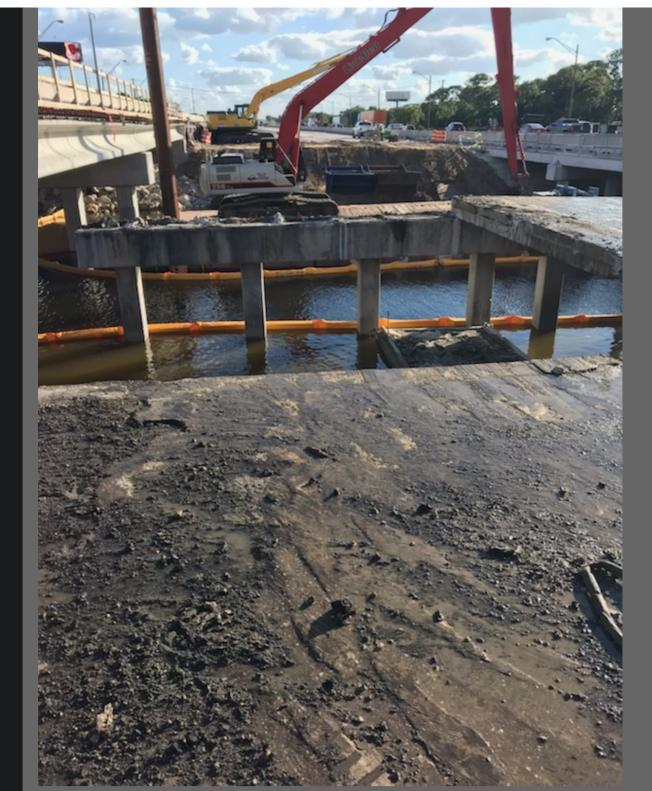
Due to the active waterway below & the multi lane expressway on both sides of the bridge, the removal was performed using specialty wire saw concrete cutting, torch cutting from barges & the use of deep cutting concrete saws.
